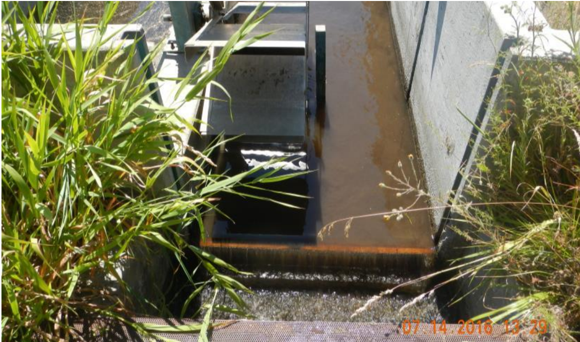
Photo 7. Pre-lease diverted flow measured at 0.74 cfs.
