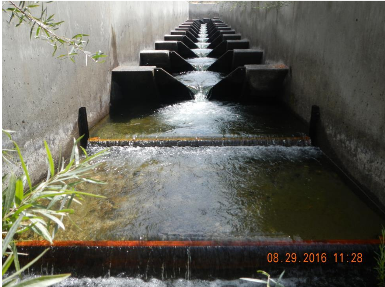
Photo 5. The full 1.5 cfs of leased water passing through the fish ladder.
