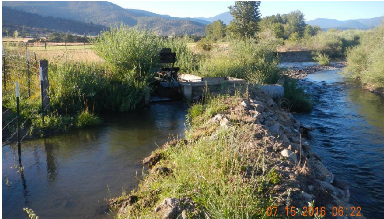
Photo 1. Flow being diverted through the fish screen (left of photo) before the lease was initiated.
